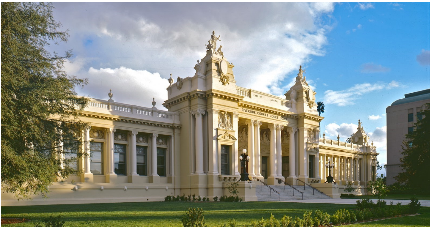
Riverside County Court House, Downtown Riverside. Digital Image. Spectra Company. http://spectracompany.com/riversidecountycourthouse .
